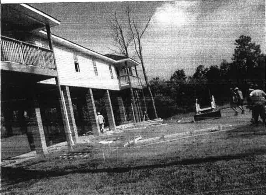
FRONT SIDE VIEW OF RESIDENCE. PICTURE TAKEN 8/28/07.
