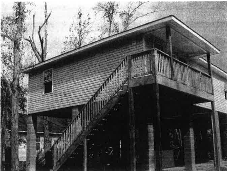
LEFT SIDE VIEW OF RESIDENCE. PICTURE TAKEN 8/28/07.
