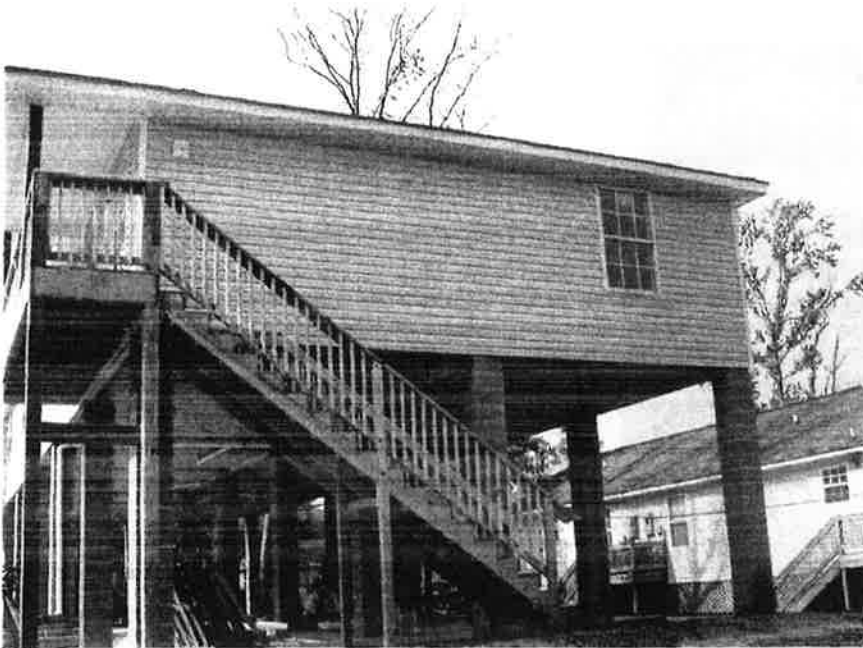
RIGHT SIDE VIEW OF RESIDENCE. PICTURE TAKEN 8/28/07.
