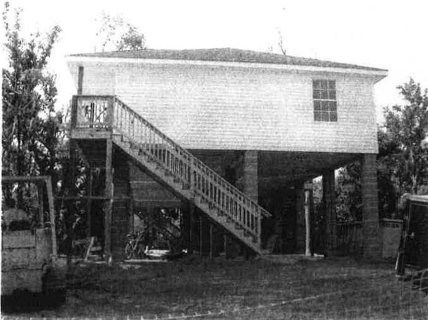
RIGHT SIDE VIEW OF RESIDENCE. PICTURE TAKEN 8/28/07.
