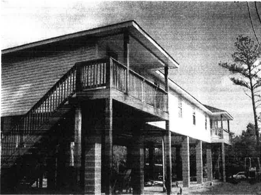
LEFT SIDE VIEW OF RESIDENCE. PICTURE TAKEN 8/28/07.
