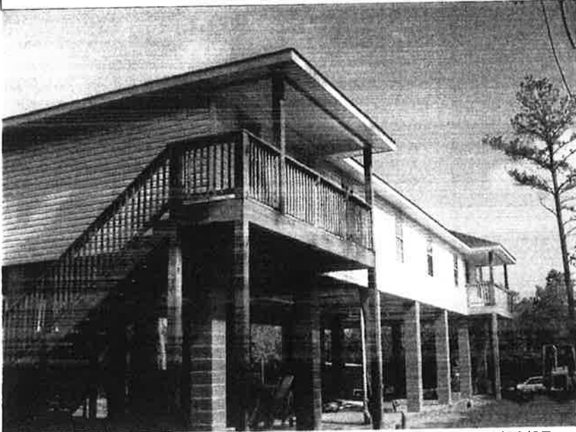
FRONT SIDE VIEW OF RESIDENCE. PICTURE TAKEN 8/28/07.
