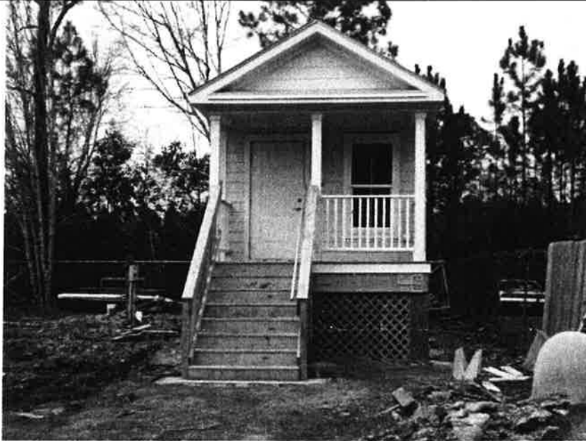
FRONT VIEW OF RESIDENCE. PICTURE TAKEN 2/16/2011.
