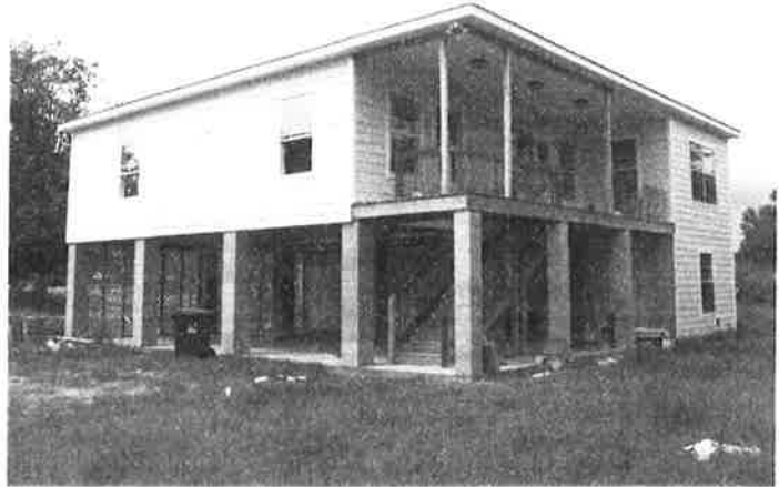
7/22/09—LOT 7, SADLER HOMES, WEST SIDE & REAR VIEW
