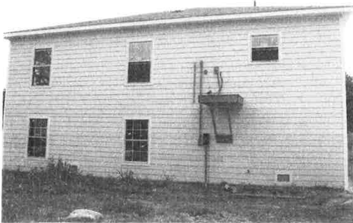
7/22/09—LOT 7, SADLER HOMES, EAST SIDE VIEW WITH RAISED AIR CONDITIONER DECK AND TYPICAL VIEW OF "SMART VENTS" INSTALLED FOR BOTTOM ENCLOSURE
