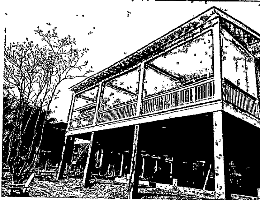
Photo Two Caption - REAR VIEW 01/02/2018
